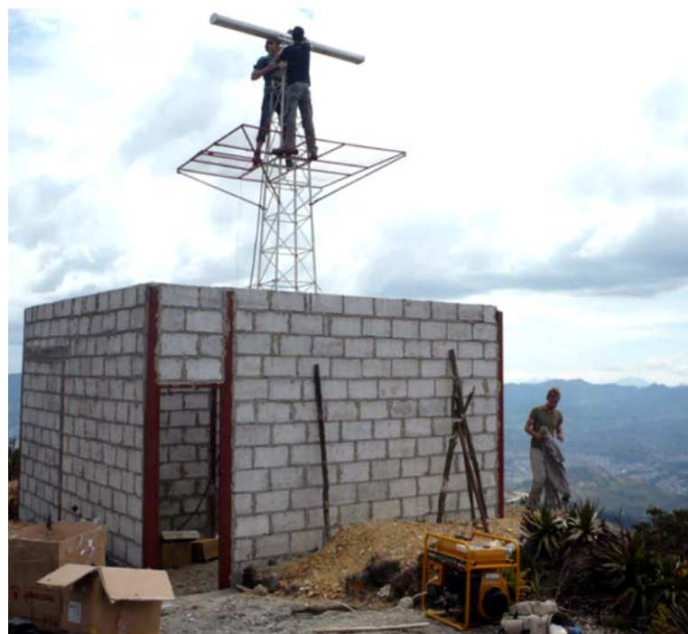
Figure 14: Radar housing for the radar at El Tiro, the mountain range near the city of Loja. The same custom-made housing will also be constructed at the other two radar sites. On the photo, the antenna for the Local Area Weather Radar (LAWR) is installed by two people on top of the radar tower. Photo: A. Fries
