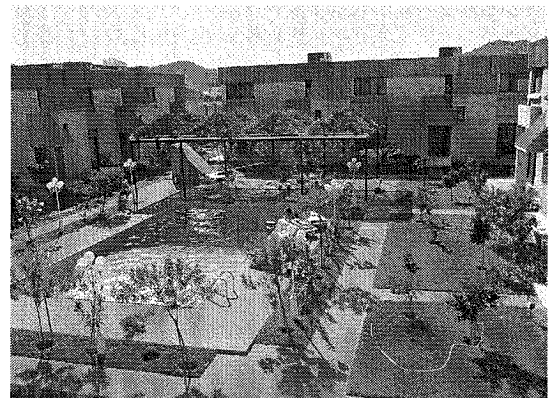
Fig. 2 Swimming-pool in a compound in Saudi Arabia
